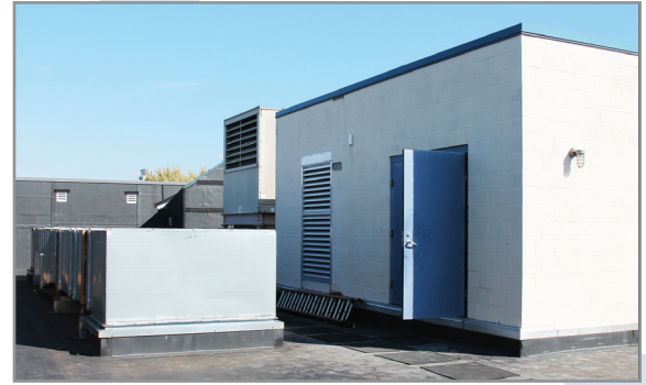
Rooftop Boiler Room
